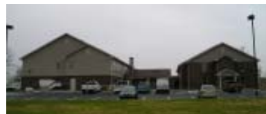
Rear View of ORR
